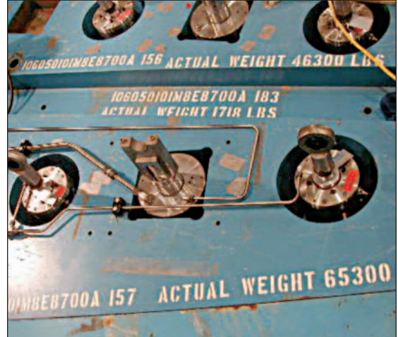
Figure 4. View of shutter top with bridge beam removed, showing the lift cylinder (center) and Sitema Safety Catchers (left and right)
